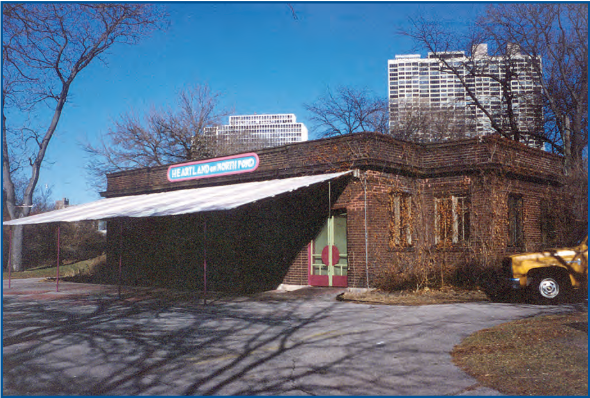
Transformed a former ice skating warming station in Lincoln Park into North Pond Cafe, a fine dining restaurant.
