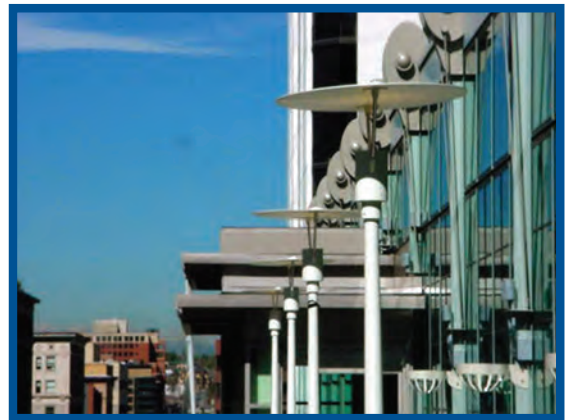
Tabor Center Exterior Detailing After Renovation
