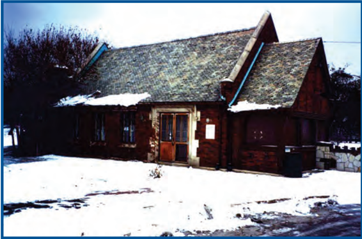
Revitalized a deteriorating storage facility at the Waveland/Marovitz public golf course into the Clock Tower Café.
